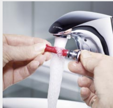
Filter reinigen/Cleaning the filter
